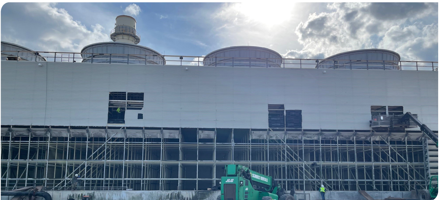
Retrofit in progress: Three cooling tower cells at TCEC are upgraded with Brentwood's ShockWave film fill.
